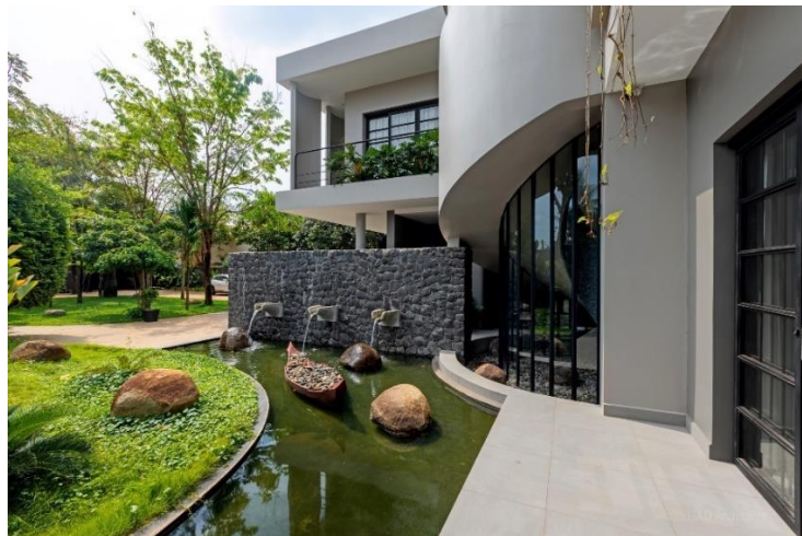
Figure 7-3: Example of integration of water feature to create microclimate surrounding the building, source: UAD Architects.
