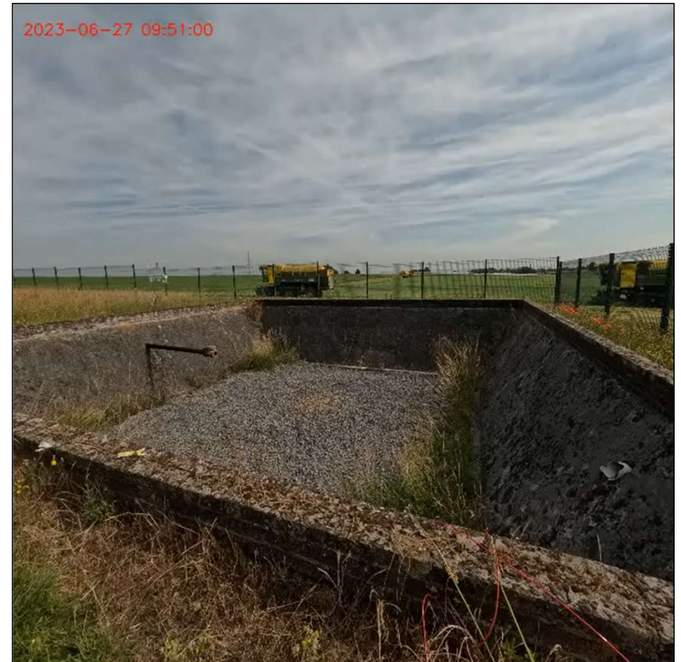
Infiltration tests in the Kemexhe basin, by Robin Glaude
