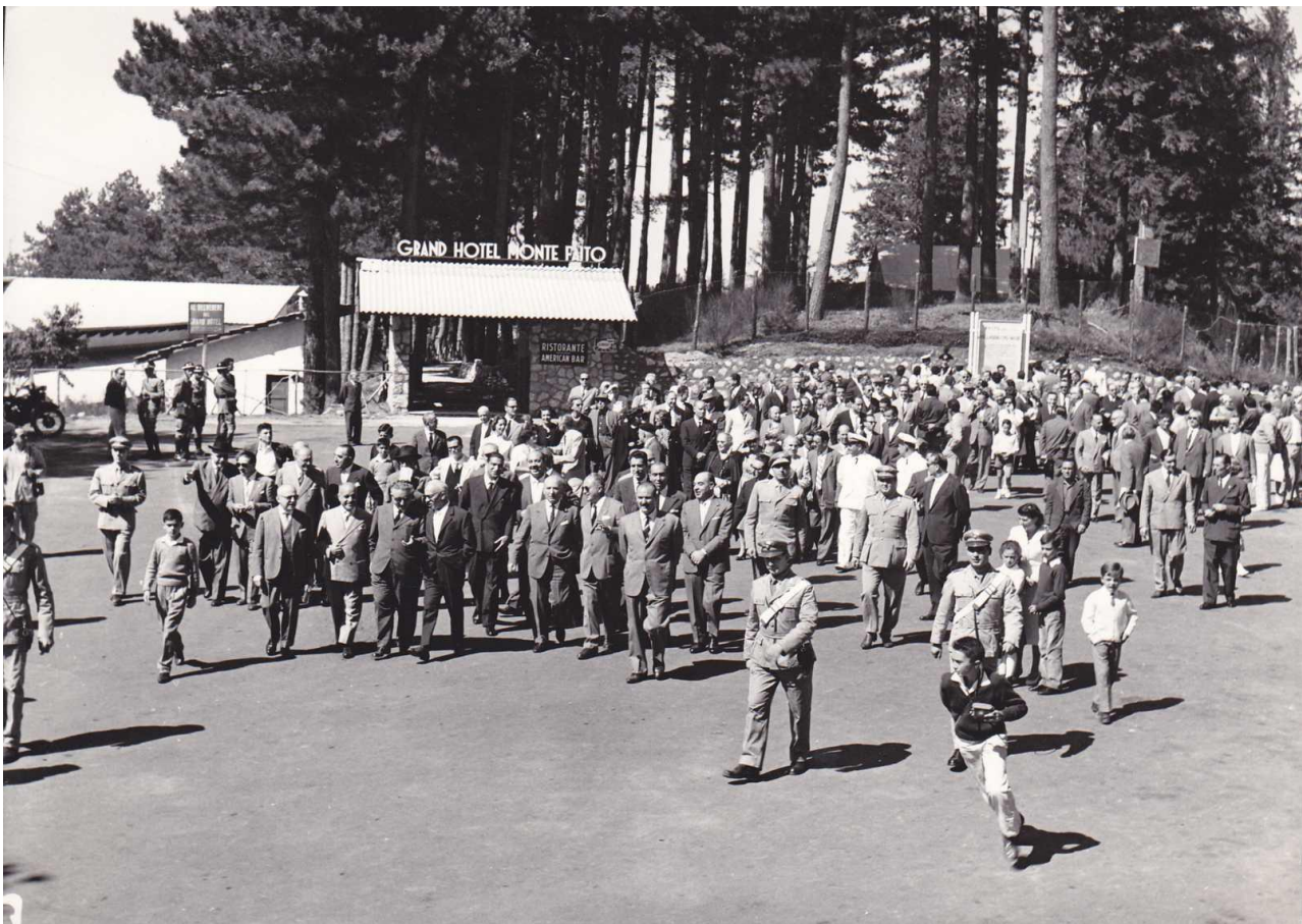
Figure 11. Historical picture of the arrival of the cablecar (Source: Profaito).
