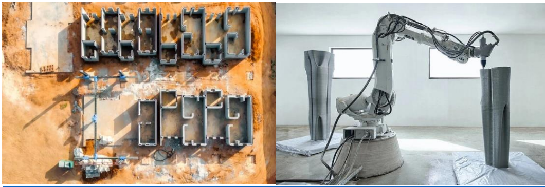
Figure 12 , left. Print ten housing units in Kenya, https://shorturl.at/sEQRZ [20]
