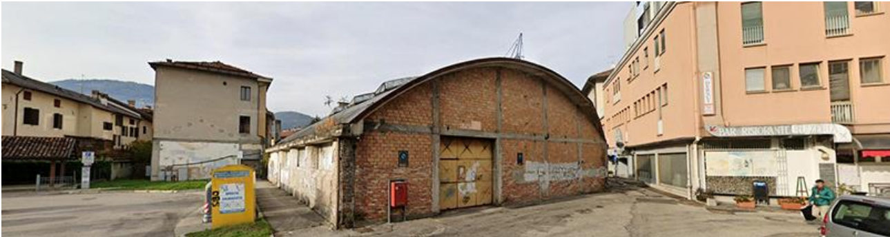
Figure 7. Piazzale della Lana, view from the south-east, current state. In the centre is the abandoned building with barrel-vaulted roof.
