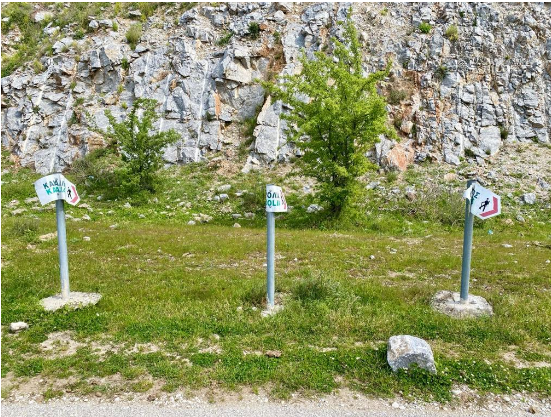
Figure 9: photograph taken by the author on March 2024, Walking signs that were damaged by the storm
