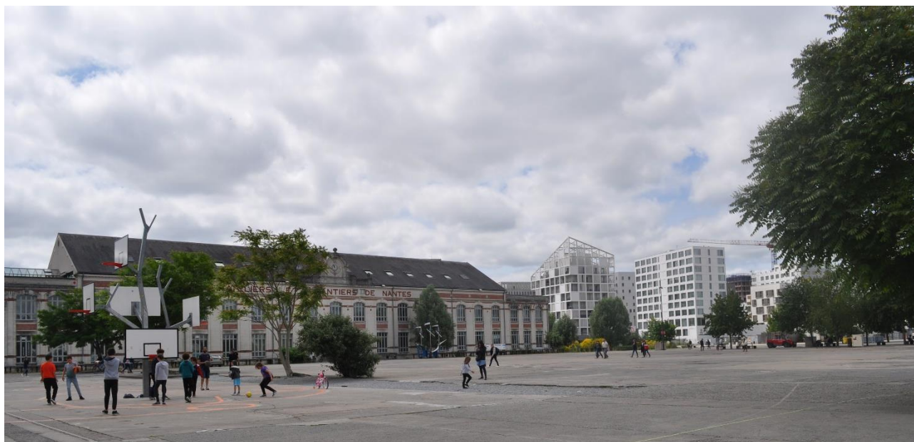
Figure 3. The transformation of the industrial urban landscape of the Ile-de-Nantes, reconverted industrial buildings, housing units and tertiary activities, Source: Varvara Toura, 2019
