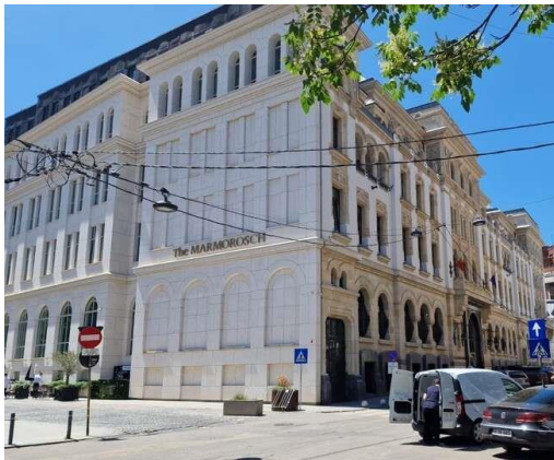
Figure 12. The Marmorosch Hotel Doamnei Street
