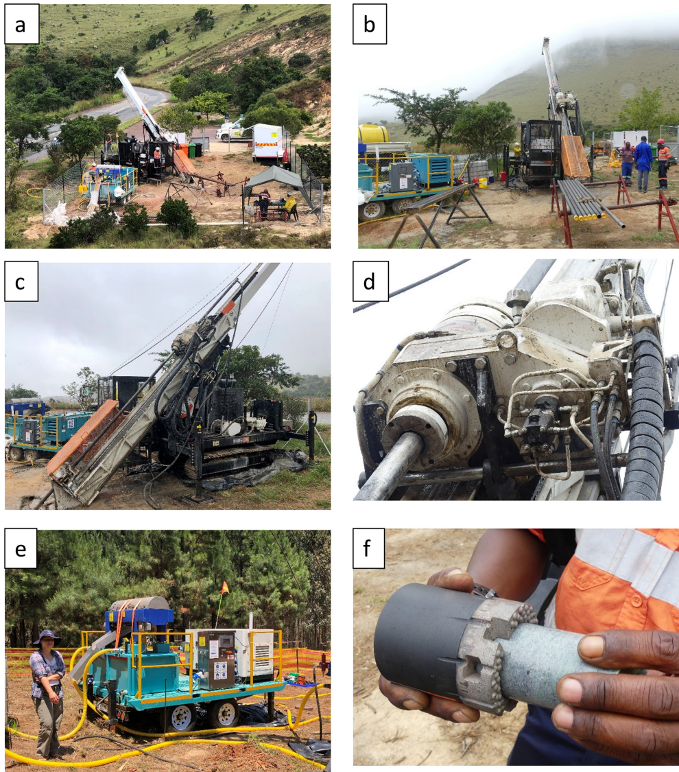
Figure 7. Drilling setup at Site 2. (a) Overview of the site: from left, bagged sludge, trailer-mounted Solid Removal Unit (SRU), drill rig MDX317, and the tressels and workbench for the drill pipes, tented work area, and storage trailer. The entire site is fenced. (b) Site overview. (c) Track-mounted drill rig. (d) “Top drive”. (e) SRU. (f) Rotary drill bit with a piece of core.
