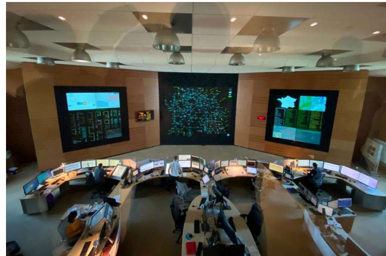
A picture of the national control centre of RTE, the French Transmission System Operator (TSO).
