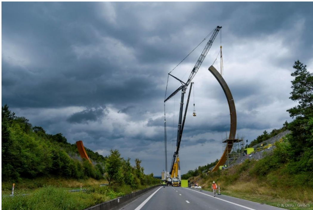
Figure 1. The “Arc Majeur” during erection
