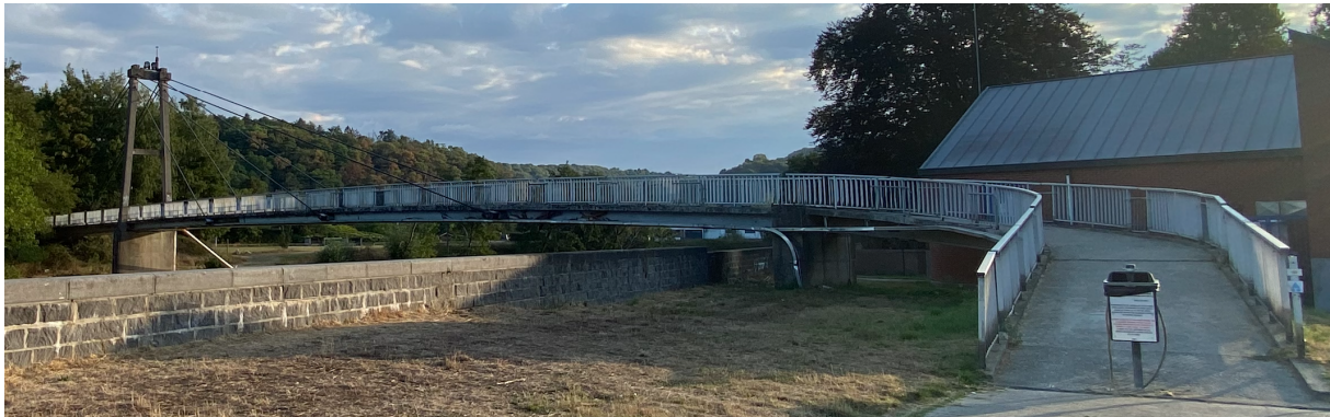
Figure 3. Picture of the Tilff cable-stayed footbridge
