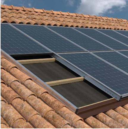
Figure 6: Solution required by the PIT and in the variant: integrated solar panels involving the dismantling of a traditional roof portion.
