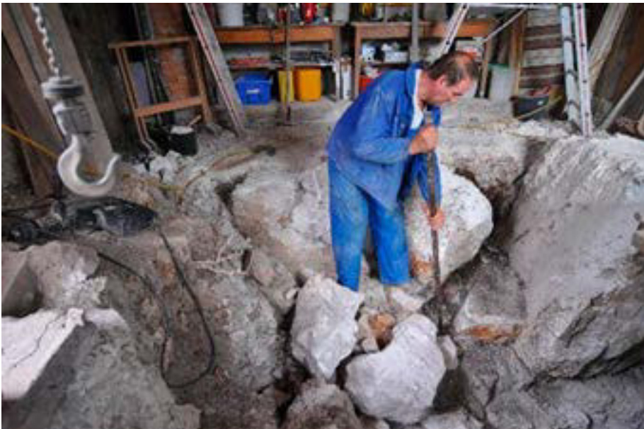
Figure 4: Room extension and work stone extraction, photo Gottfried Buchegger.
