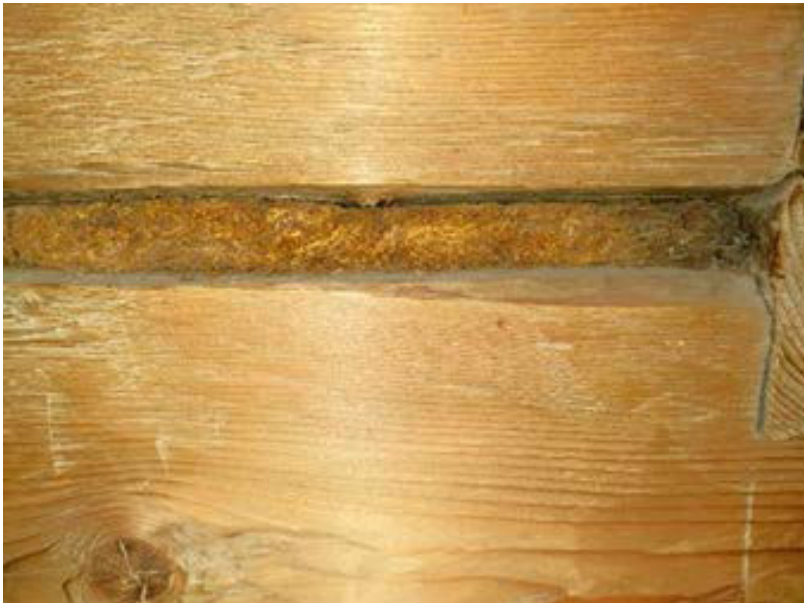
Figure 2: Beringstadel, Gosau, block carpentry 18th century. Sealing cord made of sphagnum. Condition 2017, photo: Stefanie Mandl.
