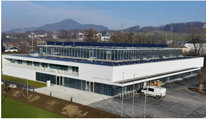
Fig.1 SPORTHALLE LIEFERING EXTERIOR VIEW (SOURCE: CITY OF SALZBURG / JOHANNES KILLER)
