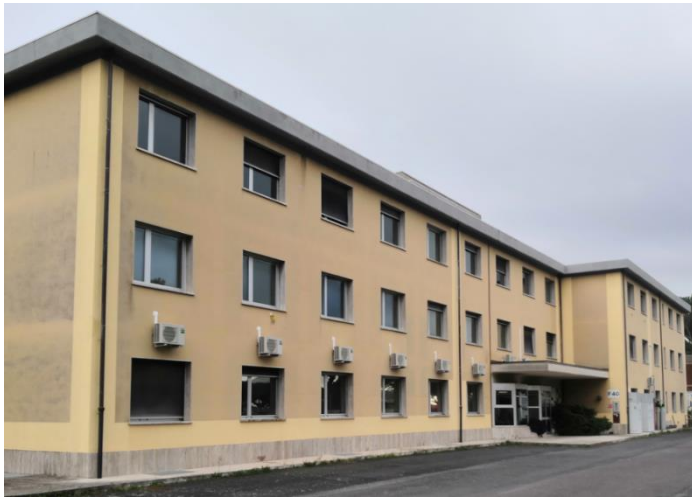
Fig.1 View of the building F40. The seven rooms of the Living Lab are those whose windows have the room air conditioner below.
