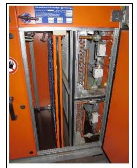
Fig.8 WOOD PELLET BOILER (LEFT) AND HEATING COILS IN THE AIR HANDLING UNIT (RIGHT)
