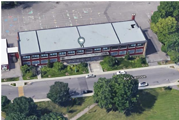
Fig.1 EXTERIOR VIEW, SOUTHEAST VIEW, SCHOOL PROJECT MONTREAL
