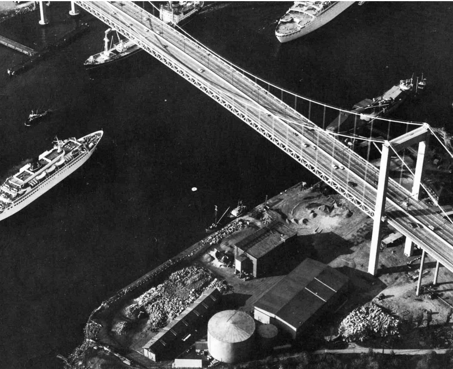
Røda Sten Konsthall (Gothenburg, Sweden) Reuse of a former boiler house, Port of Gothenburg
