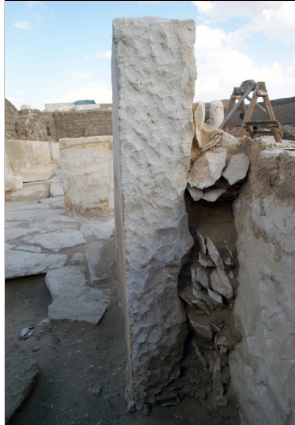
Fig. 4: An example of a hollow skin wall: the space between the limestone slabs forming the north wall of the central chapel and the south wall of the north chapel contains a rubble fill (Photo by Nico Staring/Leiden-Turin Expedition to Saqqara).
