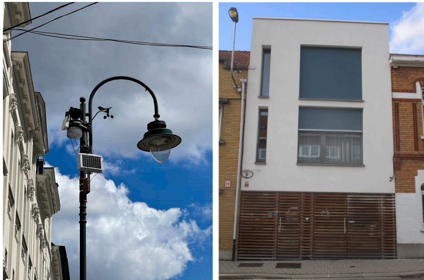
Fig. 3. Illustration of the study setup: a. weather station installed in Brussels; b. reference renovated nearly zero-energy dwelling in Brussels.
