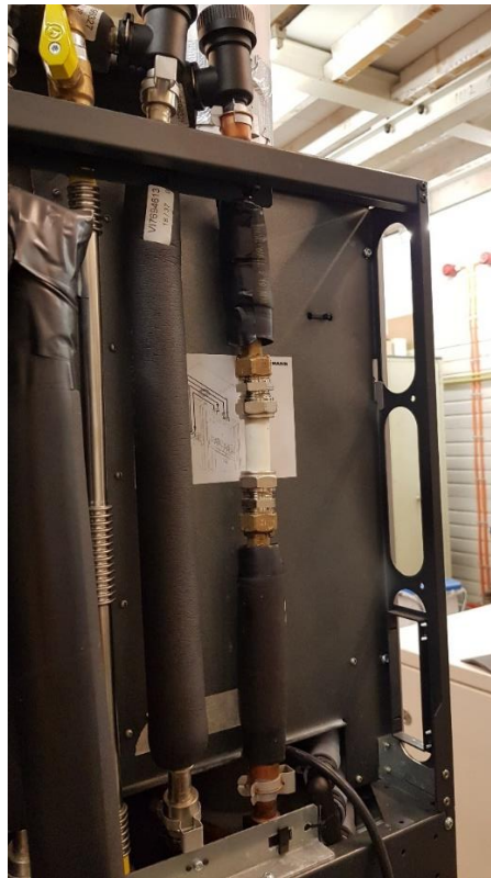
Figure 118. Boiler return line after removing the installed water meter.
