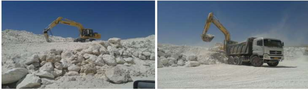
Figure 13: Gypsum extraction plant (“Photo Gallery,” n.d.)
