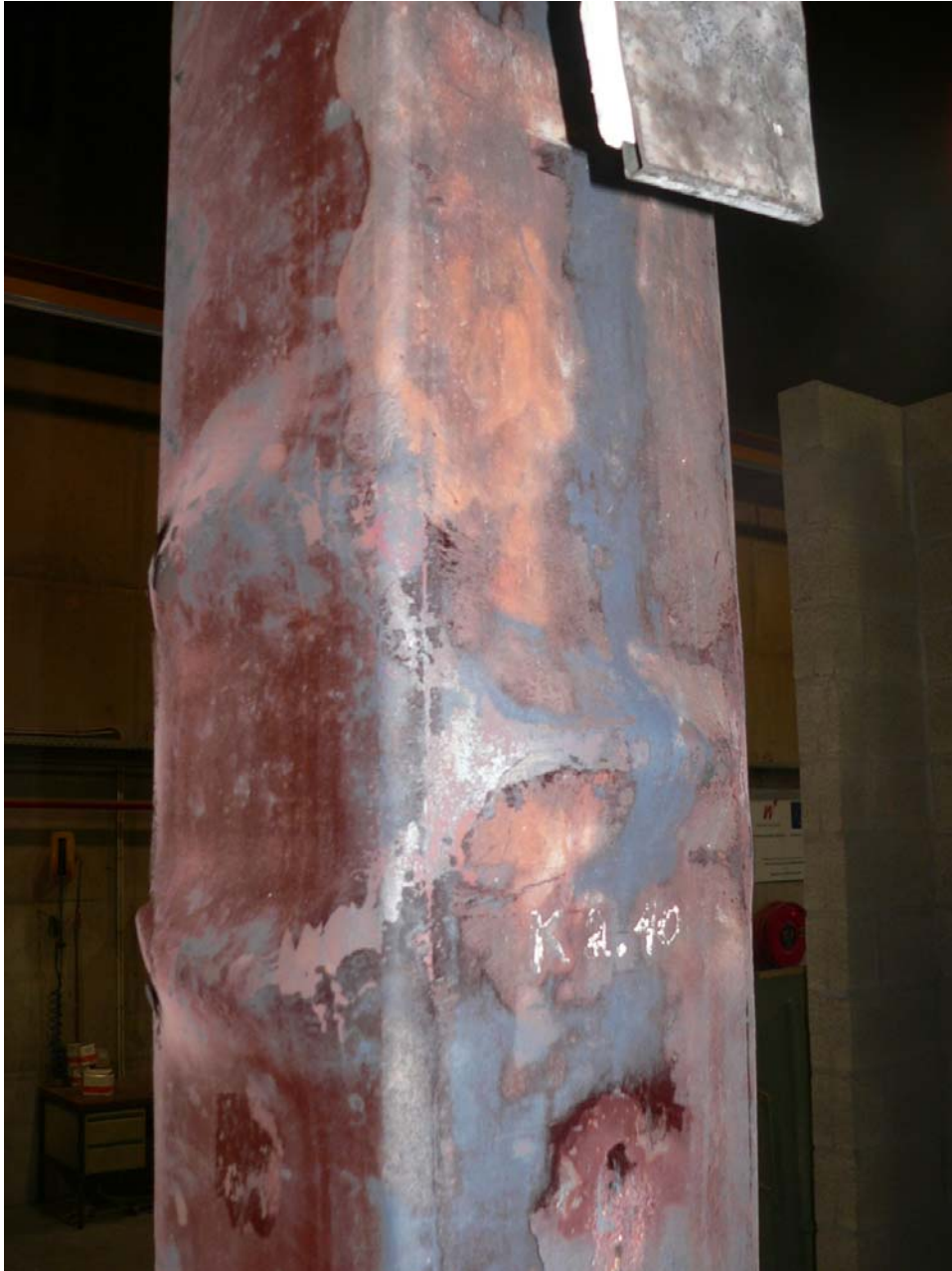
Picture A2.5. Local buckling of the test FRFC 4A
