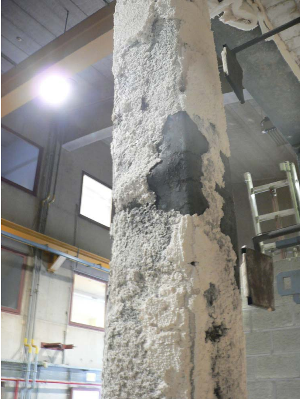
Picture A2.7. Local buckling of the test FRFC 4B
