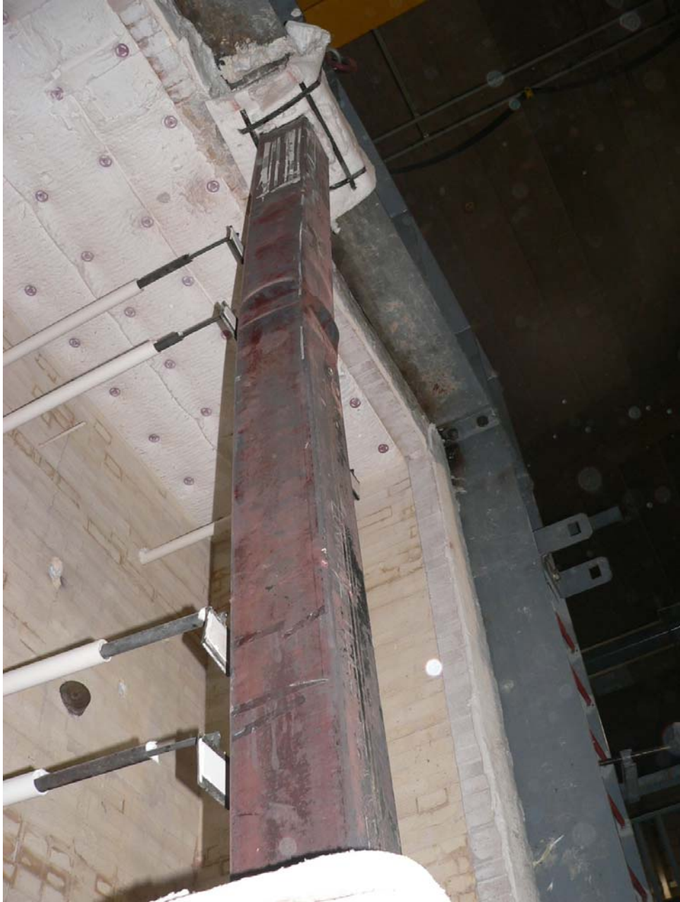
Picture A2.4. Column FRFC 4A after the test
