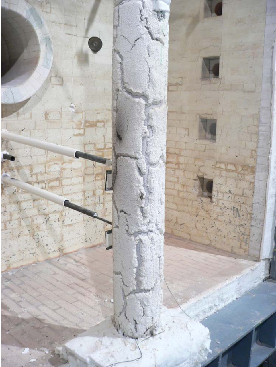
Picture A2. 3. The intumescent paint after the test of FRFC 3B
