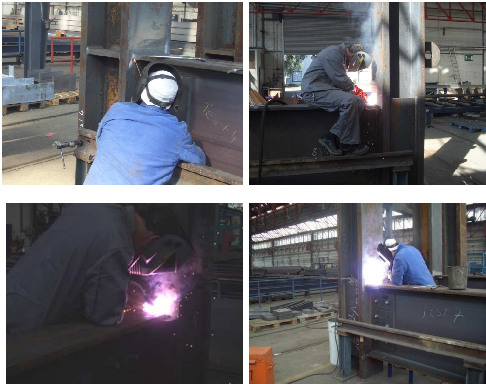
Figure 5-19: Welding of VERAPS connection
