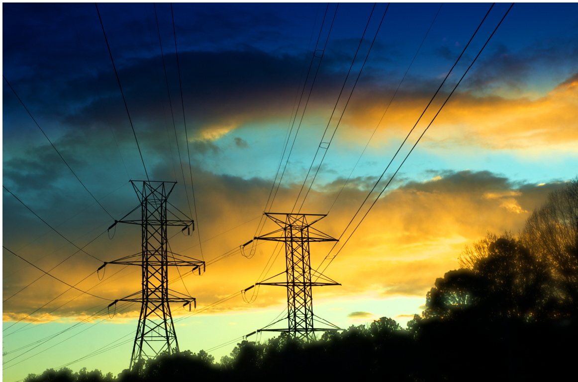
Figure 1-1. Overhead transmission lines: left – two-circuit, equipped with single conductors per phase, right – single-circuit, equipped with bundled conductors (here, twin bundle) per phase
