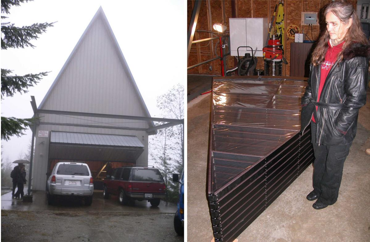
*Figure 1.23:* Left: The enclosure of the Large Zenithal Telescope located in the hills at the North of Vancouver. Right: Stored segments of mylar cover. These segments, holding  $12\mu\text{m}$  mylar sheets, go on the liquid mirror to prevent spiral waves caused by the rotation wind. Mrs Suzanne Tremblay-Hickson is seen on the photograph.
