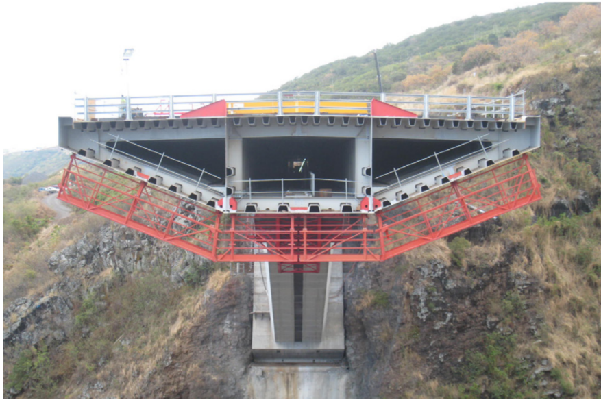
Figure 6.20: Image of the deck cross-section, during construction stage. Courtesy of Bureau d’Étude Greisch.
