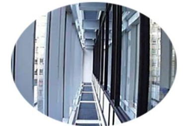
Active Ventilative Facades
