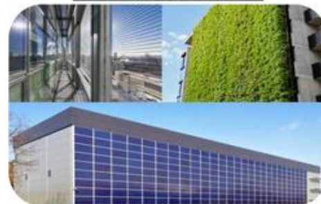
Solar active facades
