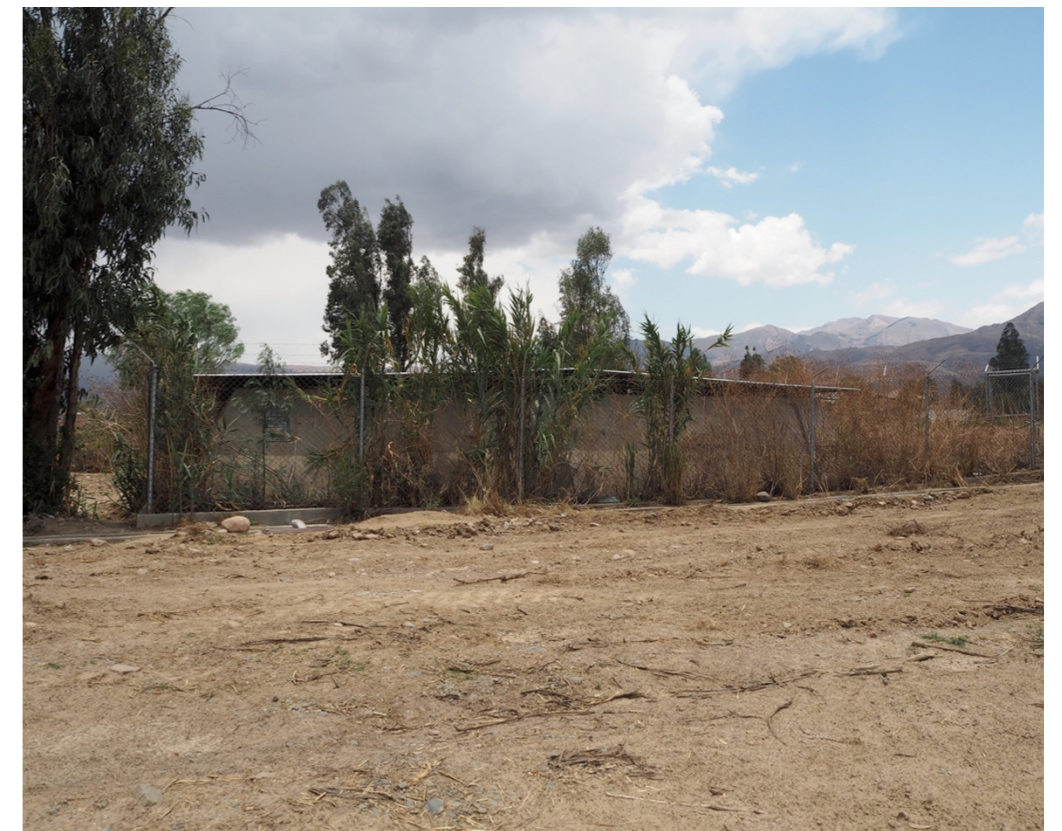
146. 147. The two collective water tanks in San Jorge A
