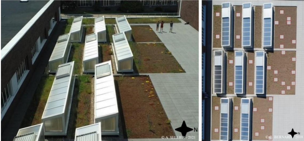
Figure 3-1 : The studied extensive green roof and the permanent plots distribution
