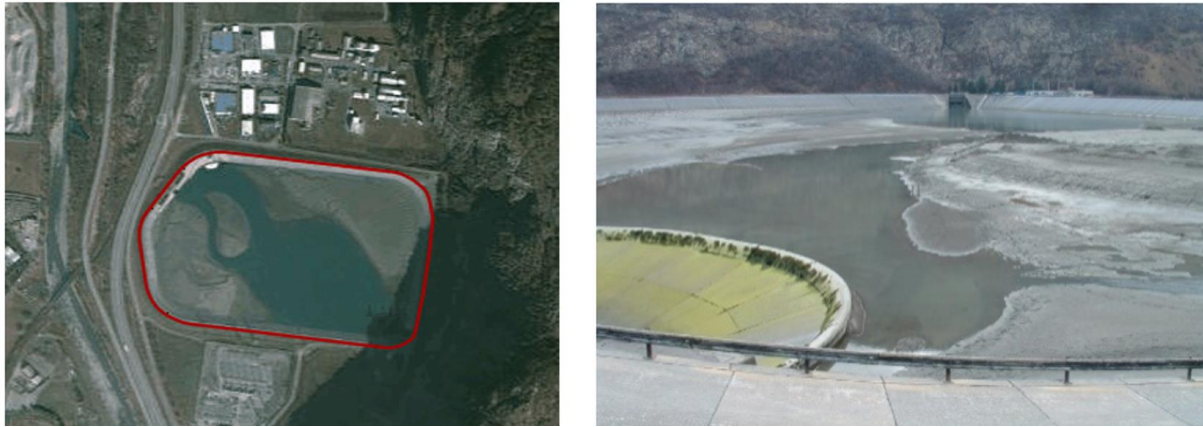
Figure 2: Longefan Reservoir (France). Aerial view (left), and reservoir after (right) sediment flushing (EDF credits)
