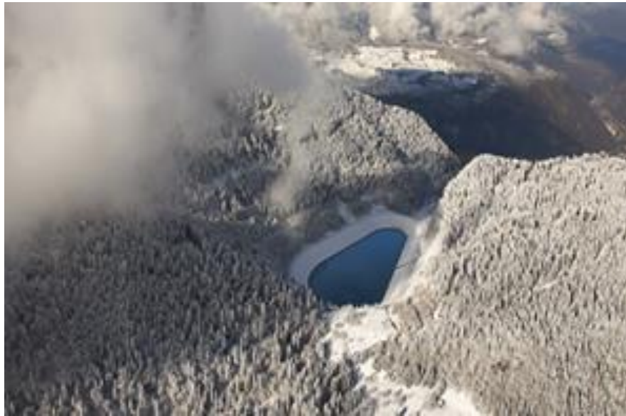
Figure 1: La Coche reservoir (France) (EDF credits)
