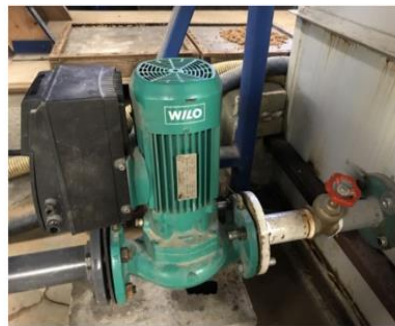
Magneto flow meter (left) and Centrifugal pump(right).
