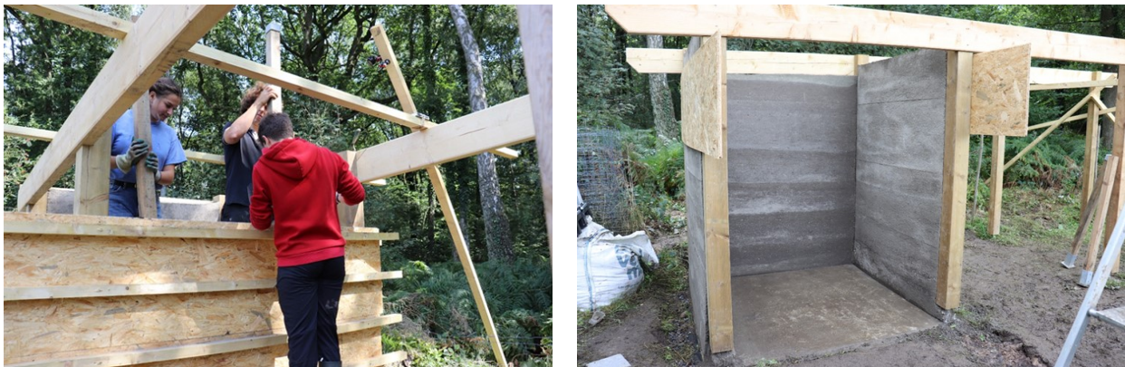
Figure 6: manufacturing rammed concrete walls with recycled fine aggregates
