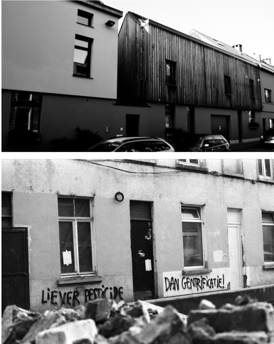
Figure 5. The renovation of terraced houses in Brugse Poort. Top photograph taken by author in 2014. Bottom photograph taken by author in 2018. Slogan in bottom photograph says “Rather pesticide than gentrification!” and most likely refers to the fact that some residents of Sparrestraat (i.e., the street where the picture was taken) took an ecological initiative to convince other street residents to refrain from the use of pesticides in their garden while around the same time 40 terraced houses in the street were being sold to a project developer.
