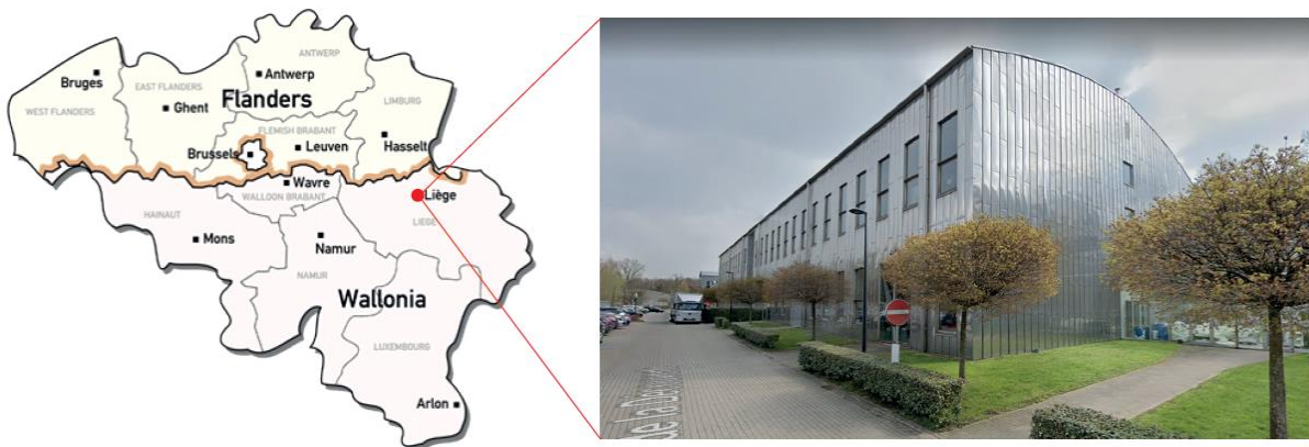
Figure 3.2 Localisation of the case study and photo of the building
