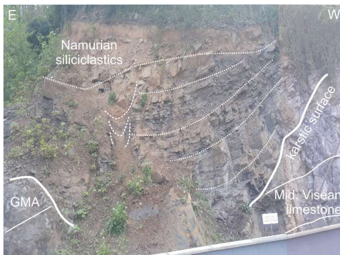
Figure 27: Palaeokarst developed in the middle Viséan limestone and filled with Namurian siliciclastics. The boundary between the two units corresponds to the erosion surface capping the Dinantian shelf. Abbreviation: GMA: Grands maladies Mbr.
