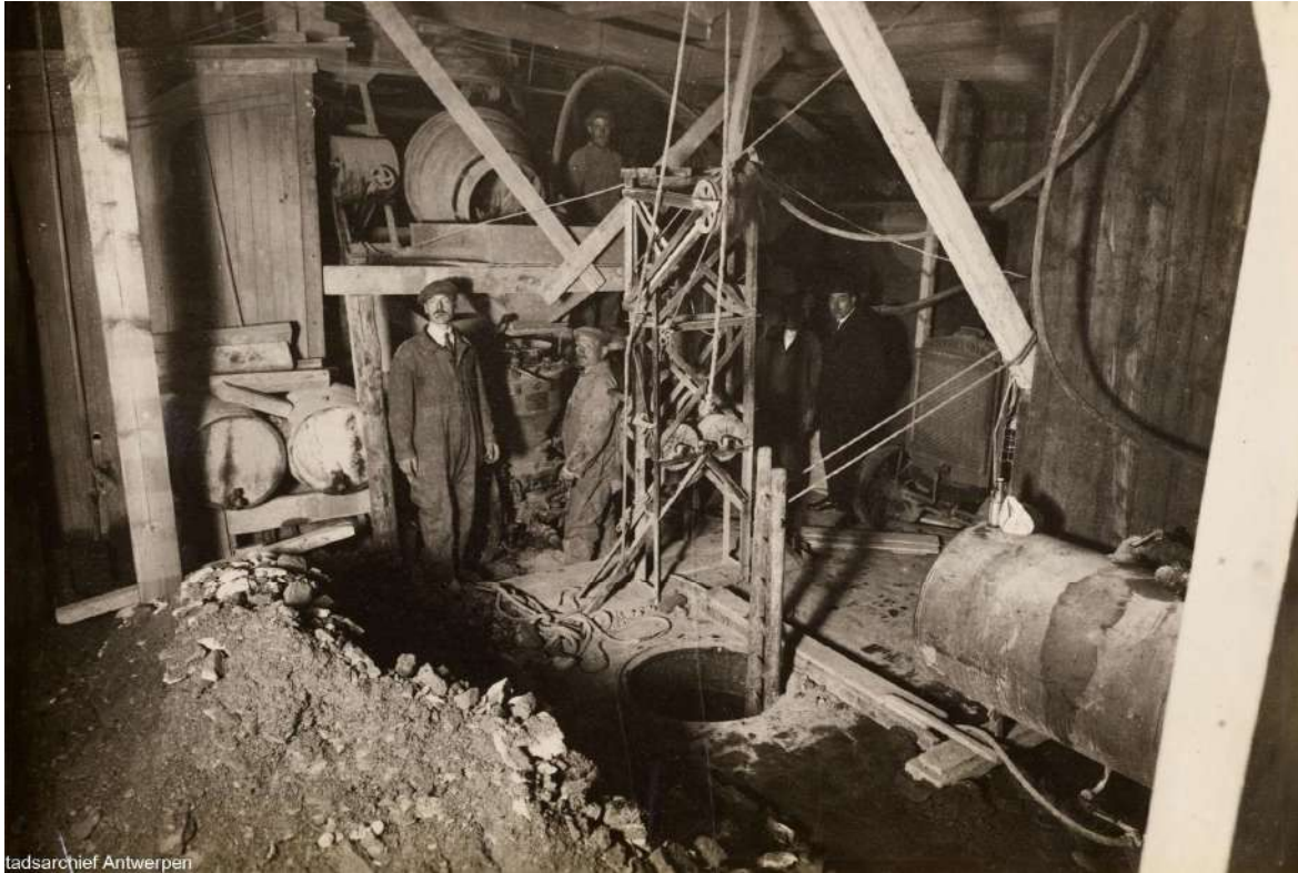
[fig.2] Betonnière et Gun (canon à ciment). Picture of the 'hold' of the ship that was used to hide machinery, dirt and dust from the public space. Source: Felixarchief Antwerpen
