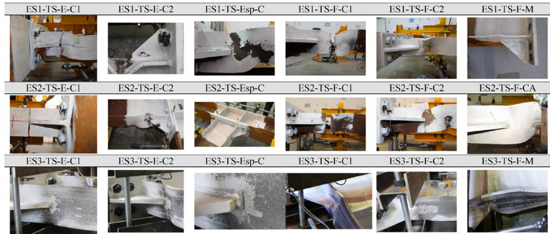
Fig. 8. Pattern of cracks in the damaged joints at the end of the tests (i.e., for ES1 and ES2 after the constant amplitude cycles at the maximum stroke of the actuator).
