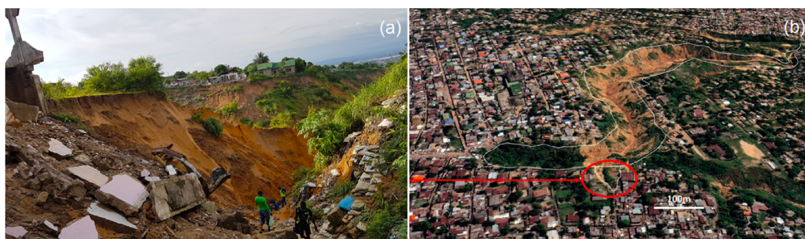
Fig. 1. Example of a new gully head that formed on the earlier existing "Laloux" gully in Kinshasa and destroyed several houses. (a) terrestrial photo of the gully head (November 2019). (b) aerial view of the same gully head (Google Earth, April 2019).
