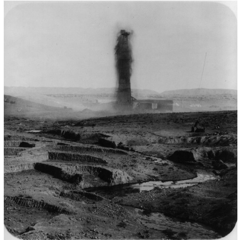
Kirkuk oil field (Iraq) in 1932. The oil extracted from this field at the time mainly benefited the United Kingdom. This is an example of energy colonialism that should not be reproduced with RREH.
