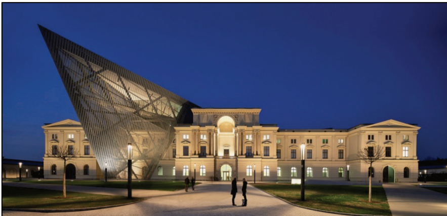
Figure 1.2: The Museum of Military History, Dresden Germany. New addition by architect Daniel Libeskind
