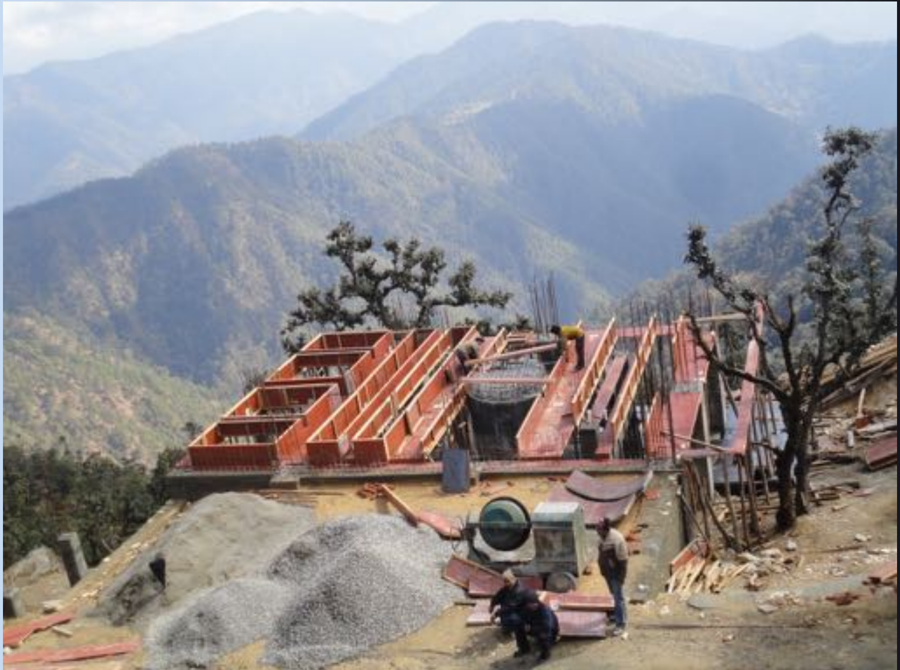
ILMT dome construction on the Devasthal site (7 February 2013)
