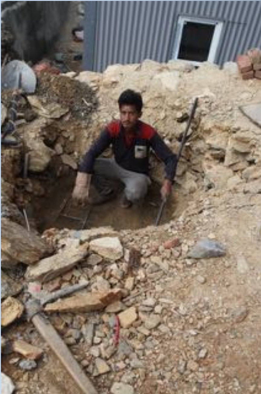
Digging 7 holes, 10 feet deep, to look for good earth grounding (June 2016)
