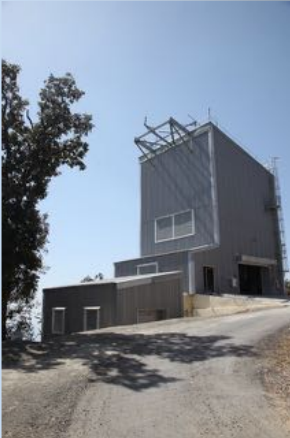
View of the ILMT compressor, control and main ILMT buildings
