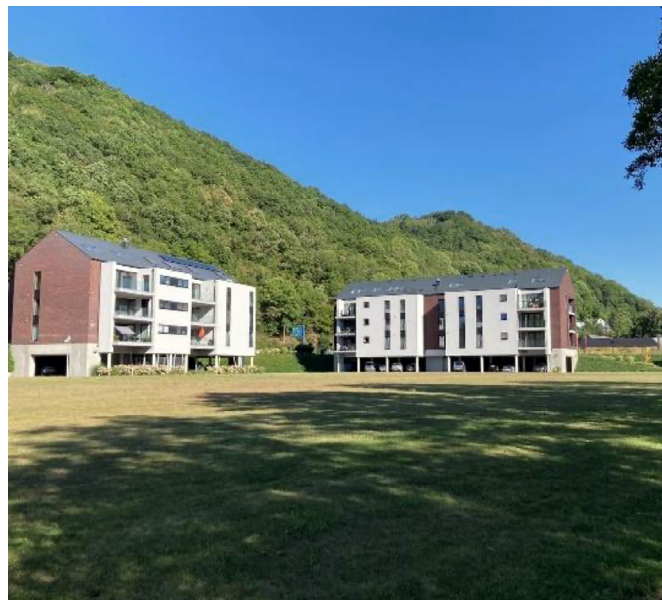
Figure 5 | Recent adapted construction in floodplains in Belgium as a part of IFRM.
