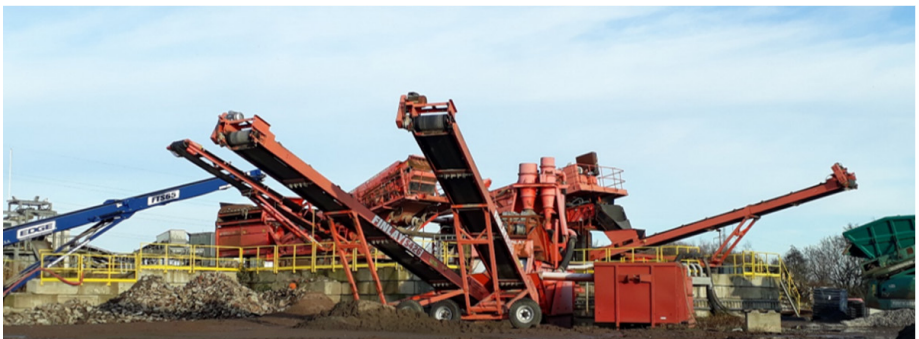
Figure 7. Picture of the final setup of the wet process installation
