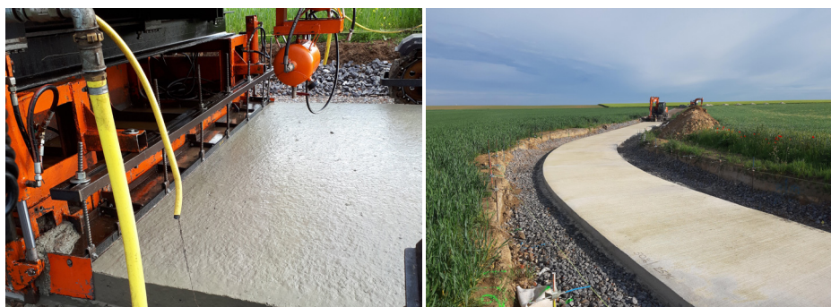
Figure 3. Regular road concrete composition placed with slipform paver
