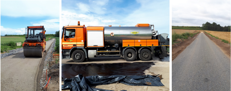
Figure 5. Construction of RCC sections, covered with single chipping surface dressing
