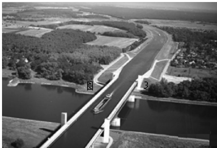
Fig. 3(a) Crossing the Elbe River
