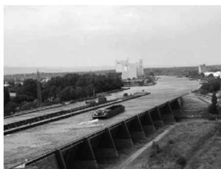
Fig. 2(c) Aerial view of aqueduct
