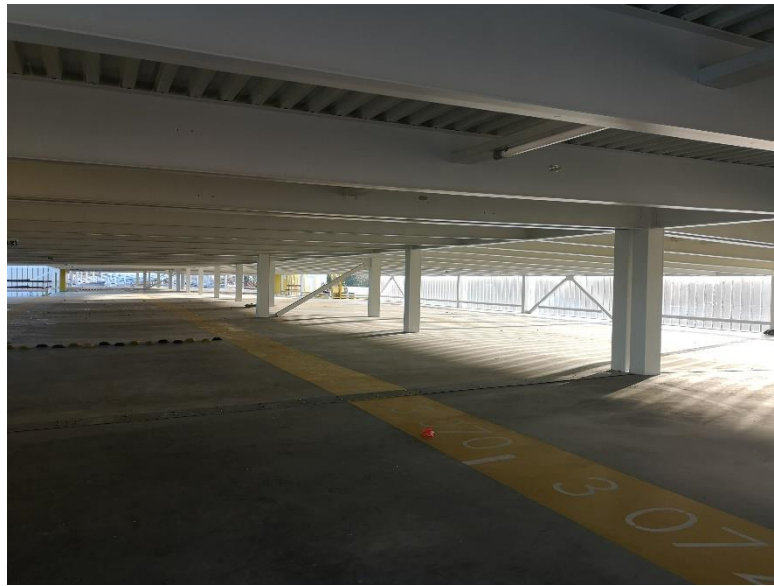
Fig.1: Composite steel and concrete parking floor in Nantes (France).
