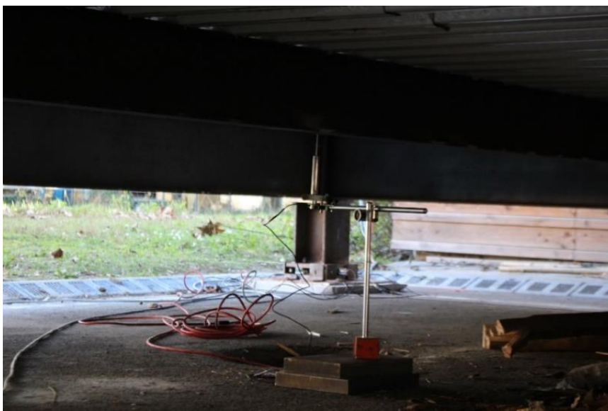
Figure 3.18: LVDT device placed below the floor
