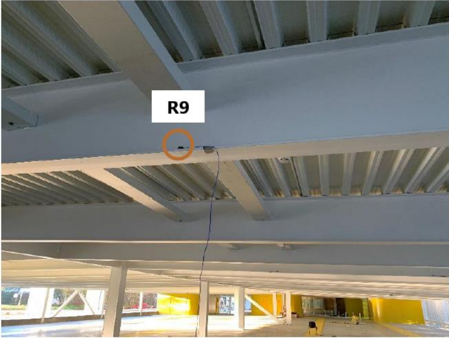
(b) Accelerometer R9 placed on a secondary beam
