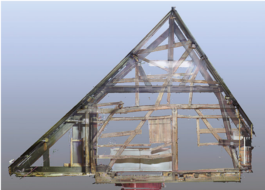
FIGURE 11 3D scan with Faro, former Beguinage of Anderlecht
