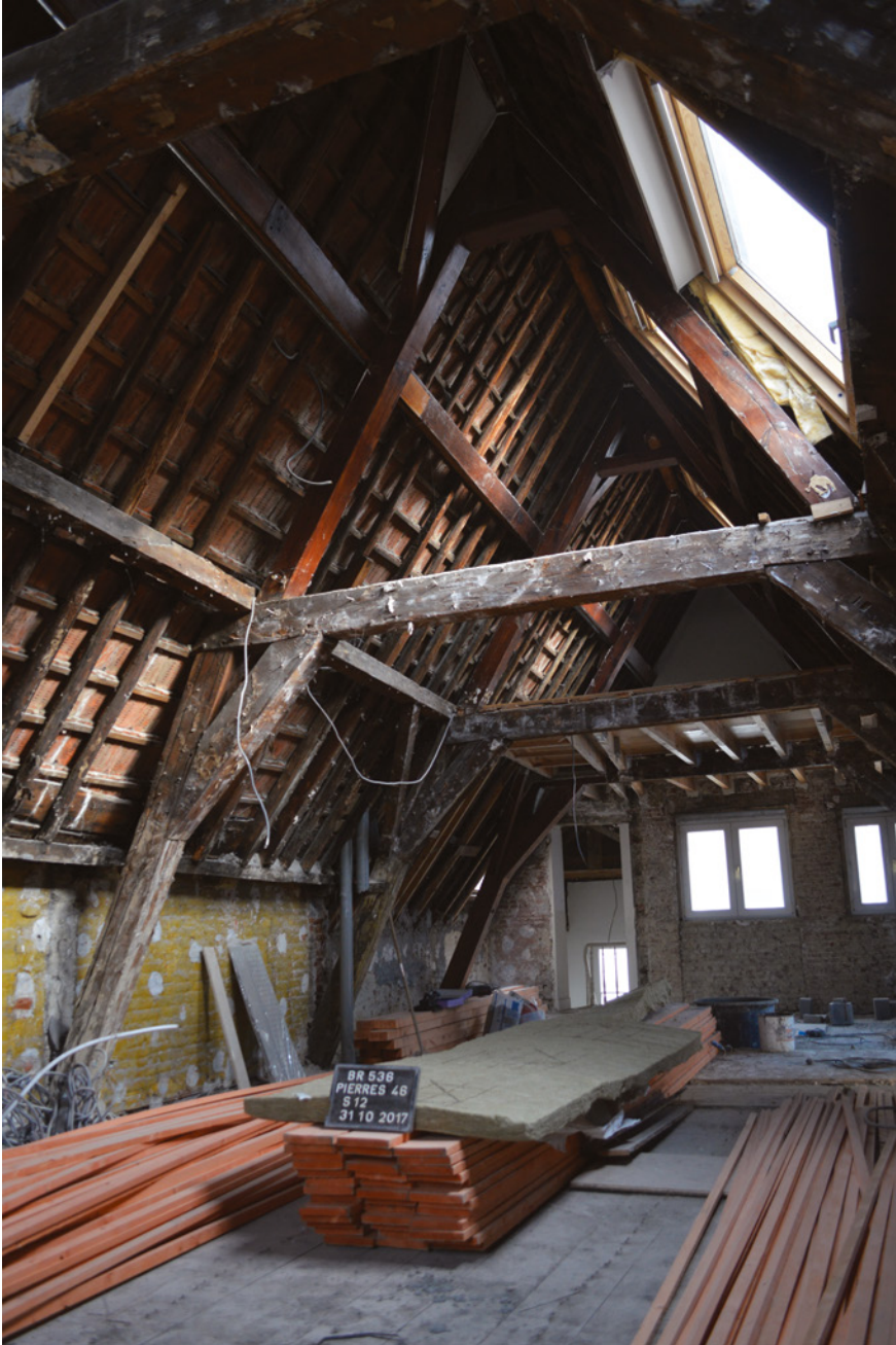
FIGURE 17 Frame in Scots pine, rue des Pierres 46, Brussels © S. MODRIE, URBAN.BRUSSELS
