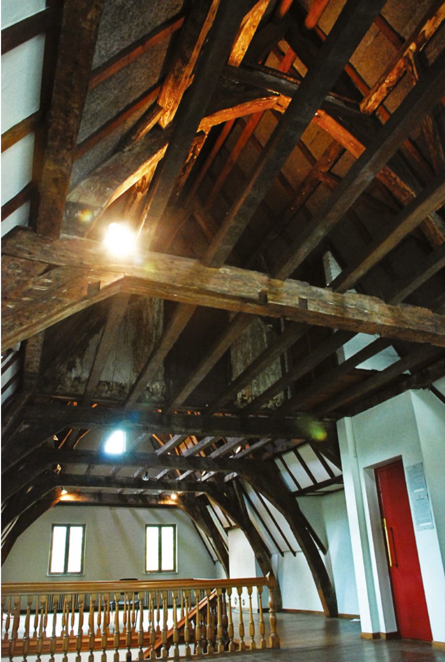
FIGURE 10 Bruegel House, general view of the attic © P. HOFFSUMMER, ULIÈGE, URBAN.BRUSSELS
