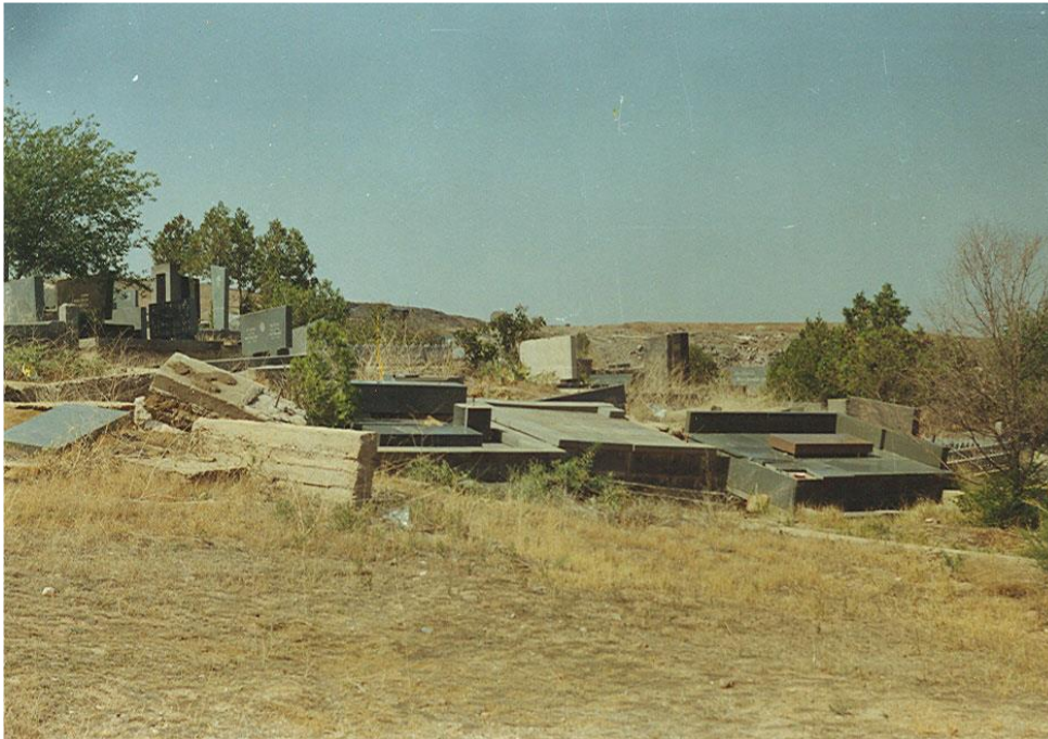
Fig. 5.16. Destroyed graves on the Nubarashen landslide, activated soon after the 1988 Spitak earthquake (from Boynagryan, 2009)
