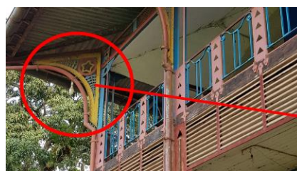
Figure 4 : decorative element used as a haunches
