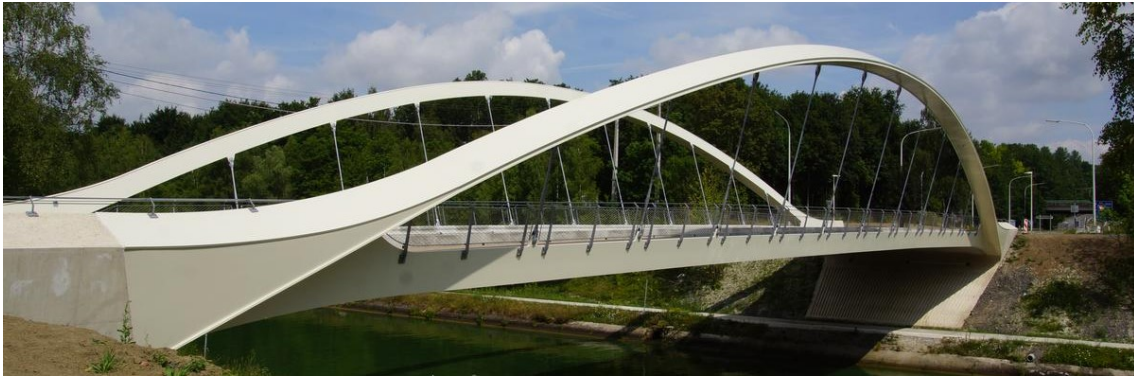
Figure 3: Photograph of the Harchies bowstring bridge, from the "Structurae" database [9].
