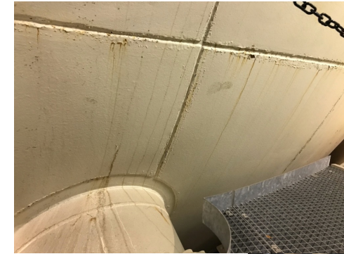
Visible signs of mundane decay, Zwentendorf NPP, 2022
