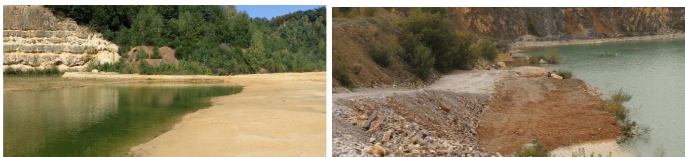
Figure 19. Softening of the slopes in the sandpit of Sablières Lannoy (left) and by addition of overburden material at les Petons (right, see outcomes in action D.2).
