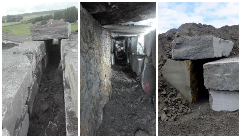
Figure 22. Construction of a bat gallery with stone blocks within a spoil heap at Carrières du Hainaut. A metal door was then installed at the entrance by the LIFE in Quarries.
