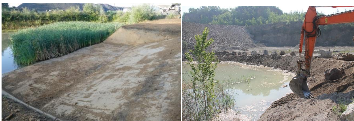
Figure 20. Sloping of technical basins banks at Milieu (Left) and Hermalle (right).
