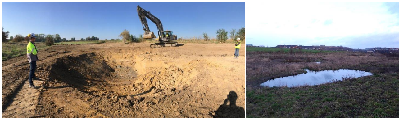
Figure 18. Before/After : Permanent pond dug and lined with clay at Clypot.
