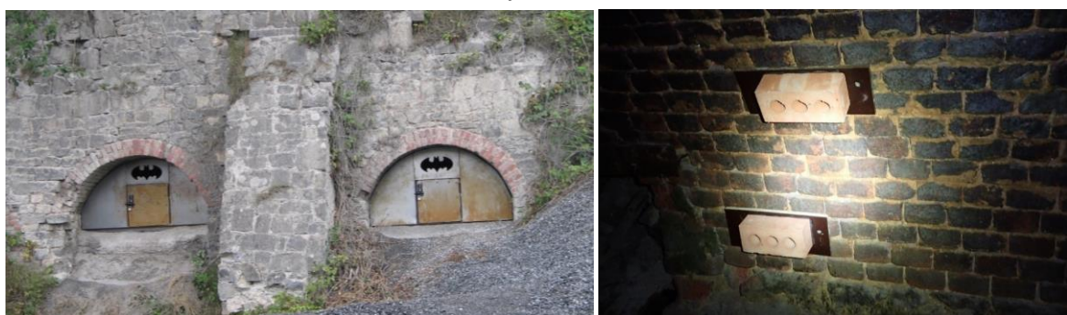
Figure 22. Construction of a bat gallery with stone blocks within a spoil heap at Carrières du Hainaut. A metal door was then installed at the entrance by the LIFE in Quarries.
