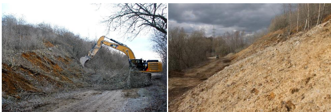
Figure 15. Sand banks with bare surface being refreshed to benefit to solitary bees and other burrowing insects Calcaires de la Sambre.
