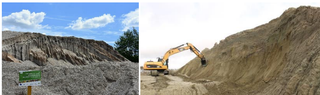
Figure 6. Vertical faces created at Carrières Les Petons (left) and refreshed at carrières du Hainaut (right) in 2016.
