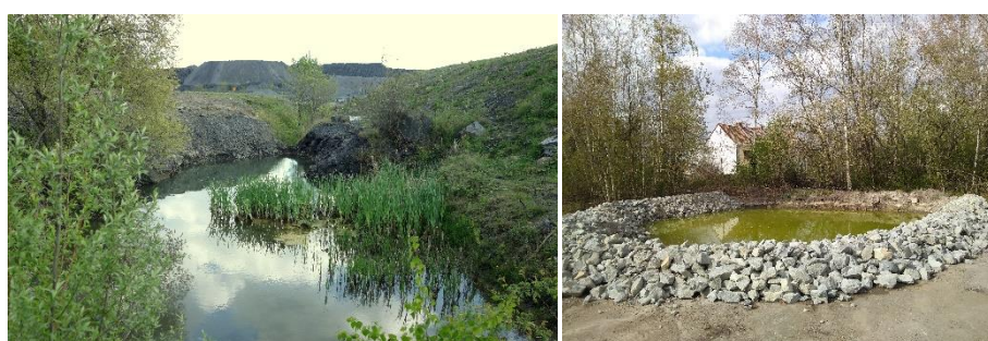
Figure 31. Permanent ponds adapted over the project at Gaurain (left) and newly dug at Ermitage (right).
