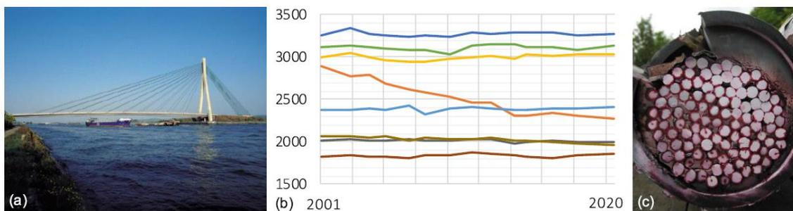
**Figure 1:** Photograph of the Lanaye bridge (left), tension variation between 2001 and 2020 in 8 instrumented stays (middle) and photograph of the cross section of a damaged stay (right)
