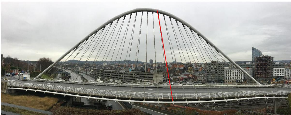
**Figure 6:** Photograph of the Observatoire bridge (stay 15 is highlighted in red)
