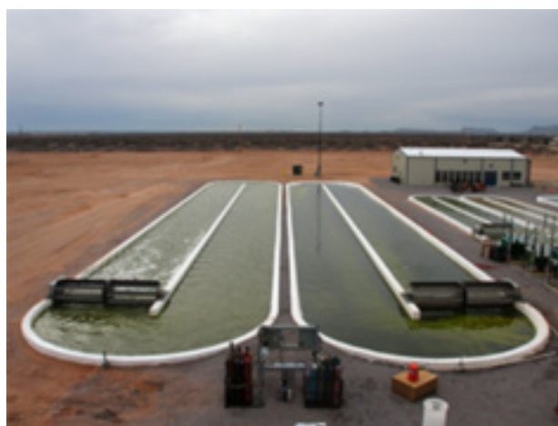
Figure 1.4 – Photography of a raceway pond for the culture of microalgae. Reproduced from (Chowdury et al., 2020).
