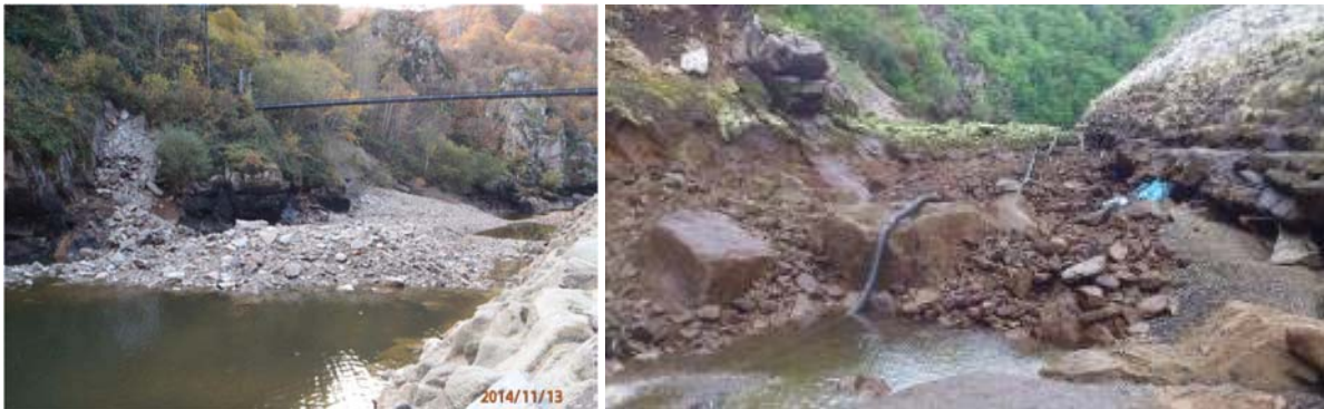
Figure 10: Deposits downstream after test at minimum operating level ( 138 \text{ m}^3/\text{s} ) (left) and scouring after test at half design head ( 200 \text{ m}^3/\text{s} )
