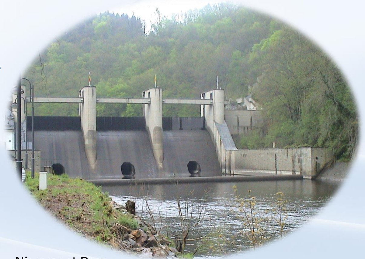
Nisramont Dam (Belgium)
