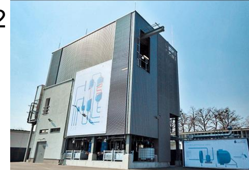
Sunfire PtL demonstration plant (top) using high-temperature electrolysis (middle) for the production of Fischer-Tropsch crude (bottom)
